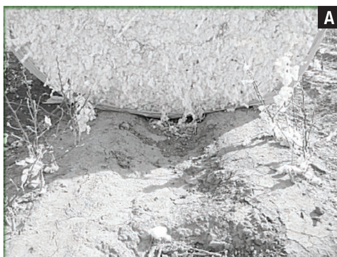
Incorrect Staging Surface
